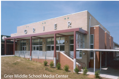
Grier Middle School Media Center
